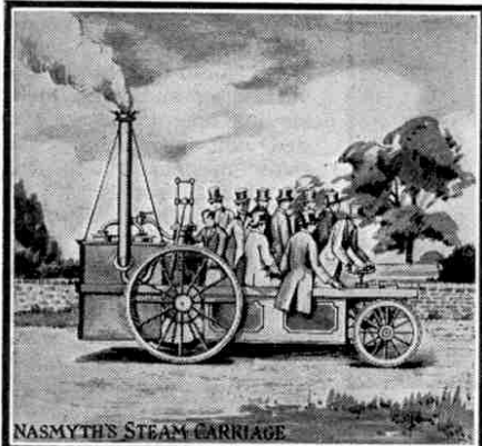
A steam-driven road carriage built about 1827 by James Nasmyth, the famous engineer. It was capable of conveying eight persons.
