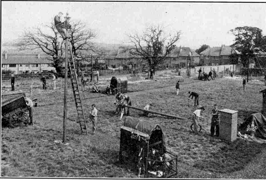
The construction park at the Dollis Hill Research Station, where outdoor equipment is tested.
