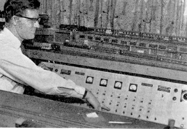
Mr. Parker operating the comprehensive control panel
