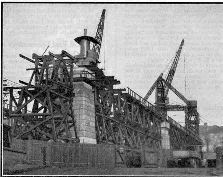
This photograph shows the progress made on the southern approach
