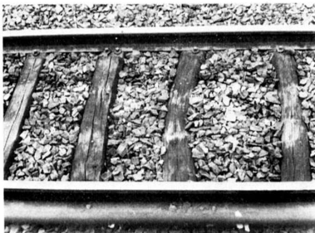
The piece of railway track at the left was photographed by John Coulson while on a visit to Northern France. This example of French permanent way between Calais and Lille startles the British eye used to ruler-straight wood or concrete sleepers at home. These sleepers at Hazebrouck are little more than squared off branches with the rails bolted down in an almost casual fashion. Despite this, all the French lines the Editor has travelled on have been notably smooth.
