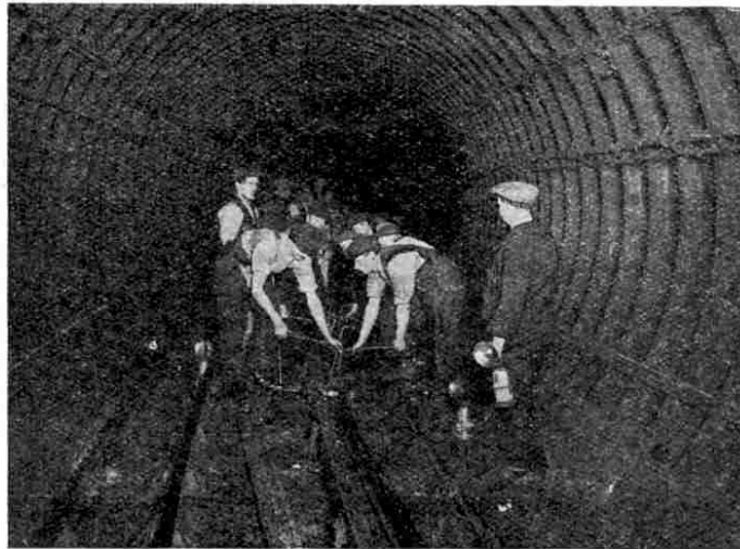
A Gang at Work on the Permanent Way
