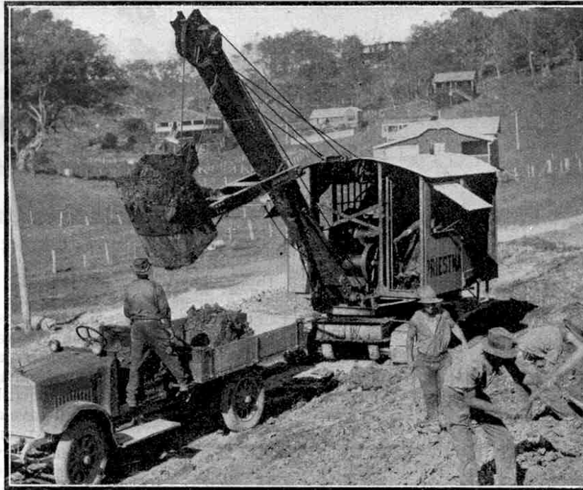
A 15-ton "Universal" Navy Shovel at work in Australia.
