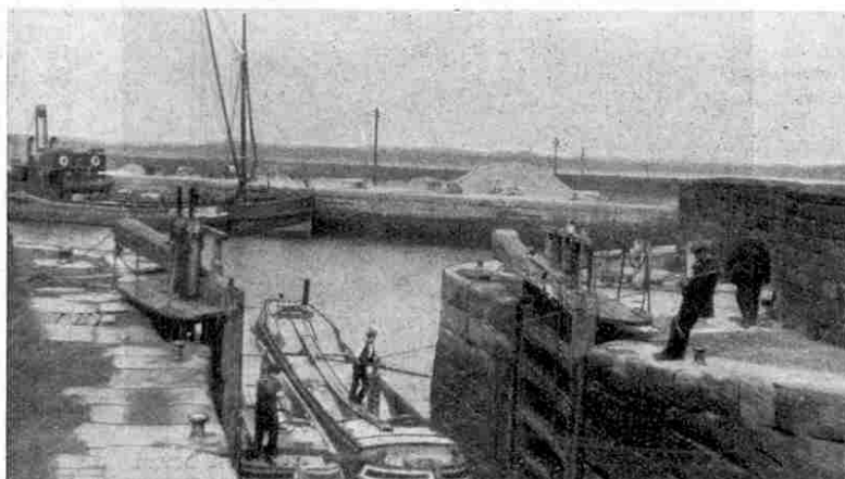
The Lock-gates opened, allowing the boat to emerge on the river level
