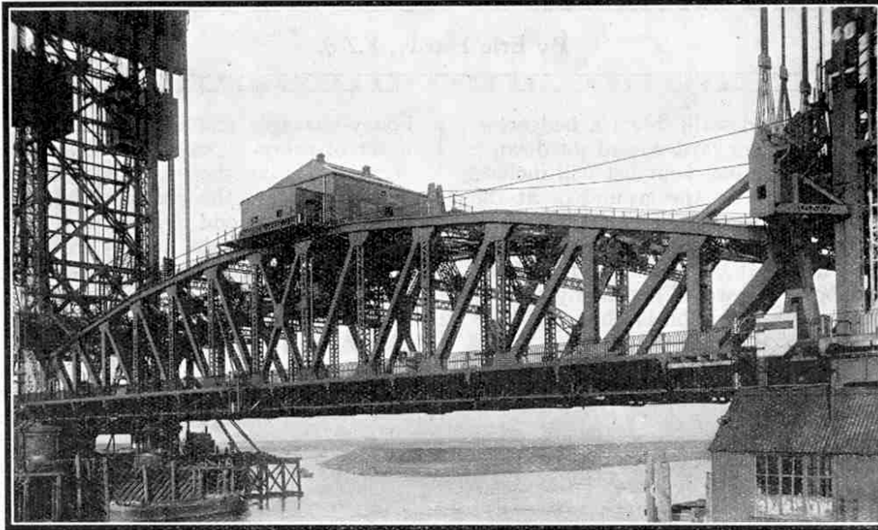
A close-up of the lift span showing the machinery house, below which the operator's cabin is situated.
