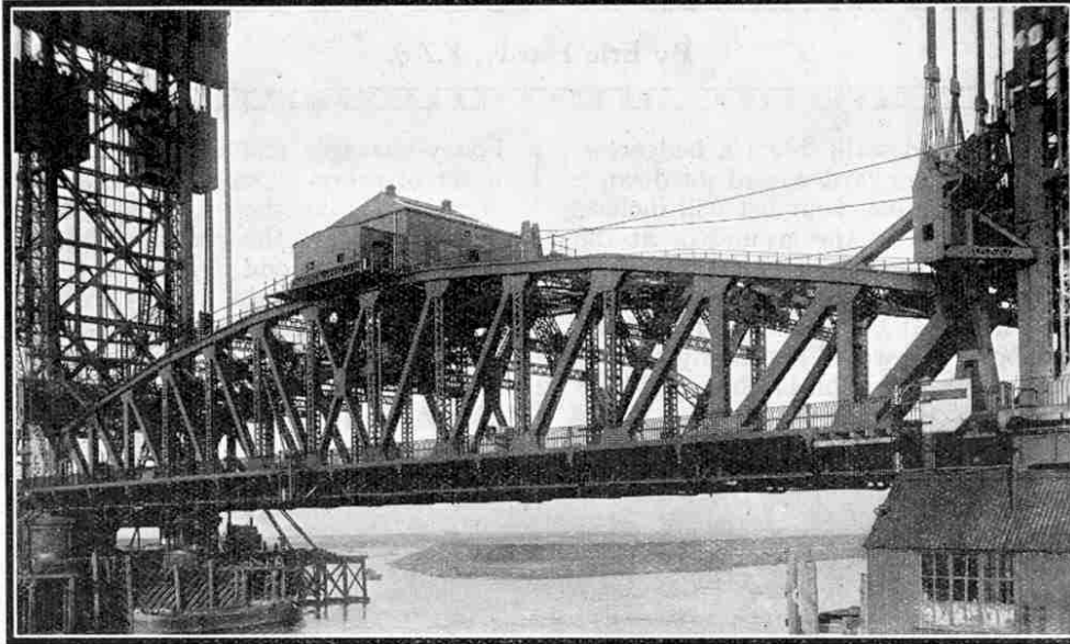
A close-up of the lift span showing the machinery house, below which the operator's cabin is situated.
