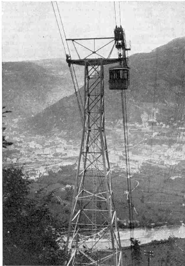
The Kohlerer Mountain Aerial Railway
