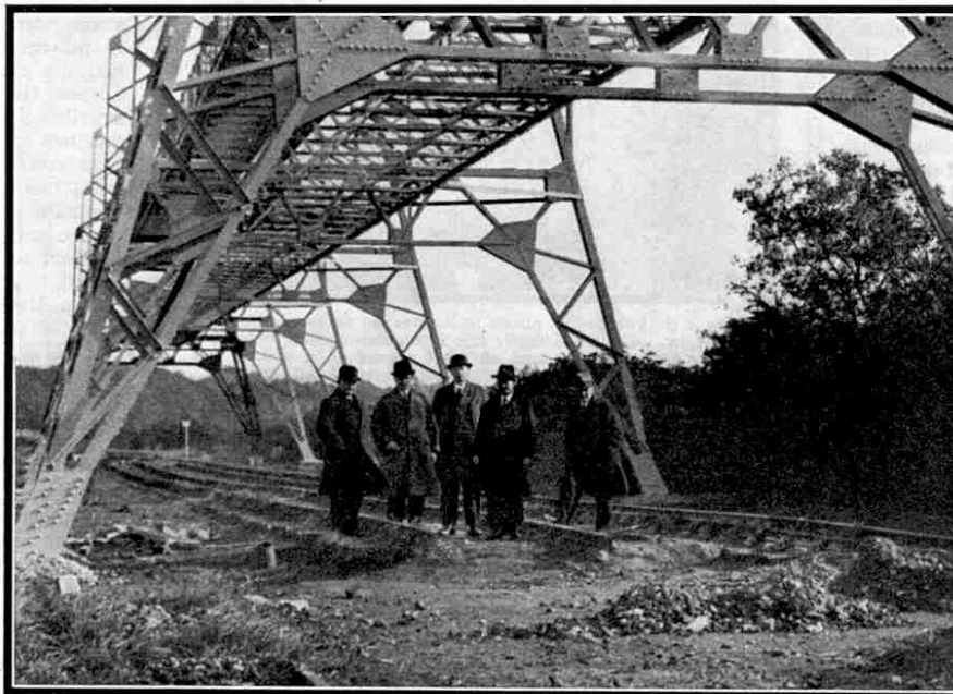
The two illustrations on this page show the test line of the Railplane erected over the track of the London and North Eastern Railway at Milngavie, near Glasgow.
