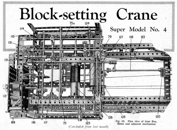
THIS month we conclude the detailed instructions for building the Giant Block-setting Crane. In the two previous articles we have dealt with the purely structural work in the model, and to complete the crane it now remains to build the gear box, crane trolley, and accompanying fitments.
