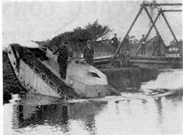
Medium D (Third Prototype) on flotation tests at Christchurch.
