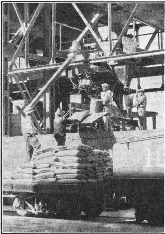
Bagging, sewing and loading granulated nitrate ready for shipment.
