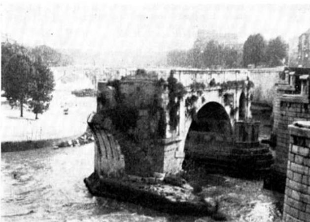
Partially destroyed by floods in 1598, and further damaged in the 19th century, the Ponte Rotto in Rome was built in 181 B.C. These remaining arches are typical Roman. In the background is the Ponte Fabricio.
