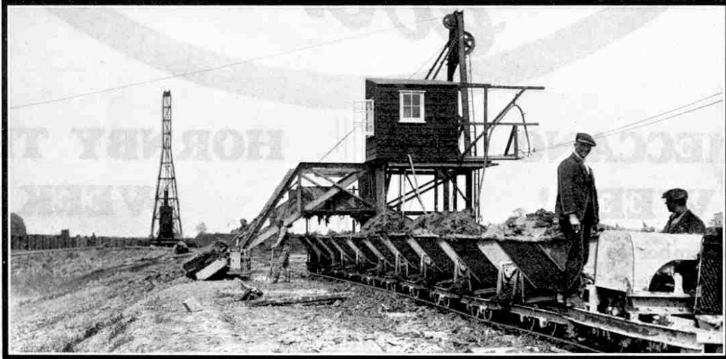
The head carriage of the Henderson Cable Drag-Scraper, with the bucket about to ascend the ramp. The tall structure in the background is a pile-driver. For this photograph we are indebted to the courtesy of John M. Henderson & Co. Ltd.
