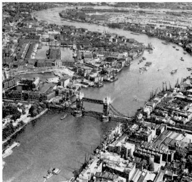
Because it can be lifted to let ships pass through, the Tower Bridge does not prevent vessels up to 10,000 tons from going up the Thames beyond the Port of London.
