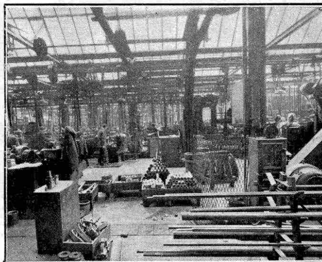
The machine shop, which has a floor space of more than 25,000 sq. ft. For the above illustrations we are indebted to "Modern Transport"
