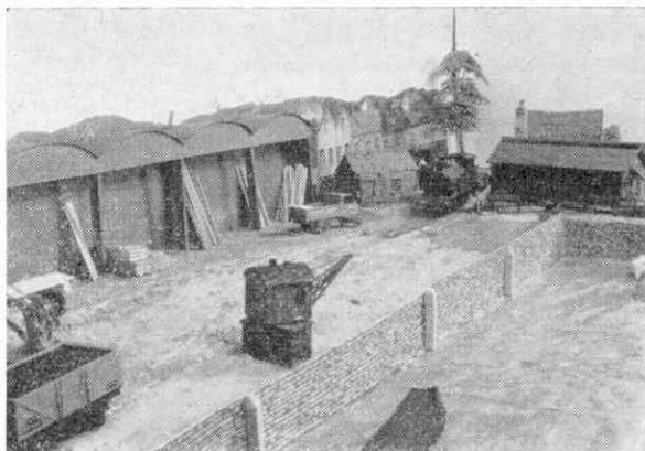
The dockside steam crane adds much interest
