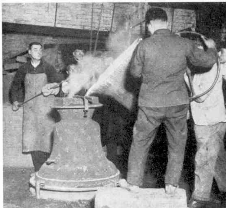
Pouring the molten metal into the finished mould to make a bell at the works of Mears and Stainbank.
