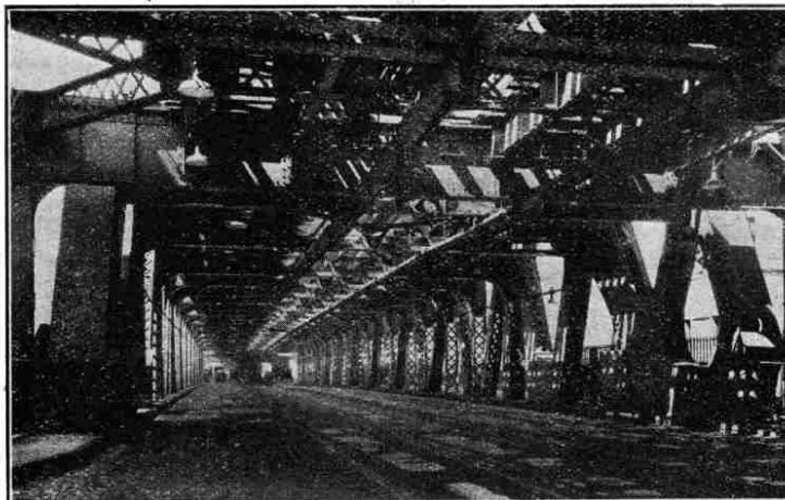
Our illustration shows a view of the lower deck of the new bridge, with its double set of car lines. The overhead railway lines are on the upper deck
